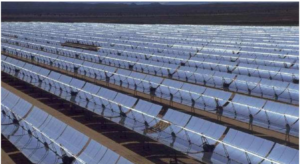
*Pictured above: A Concentrating Solar Power (CSP) facility employing parabolic trough technologies*
