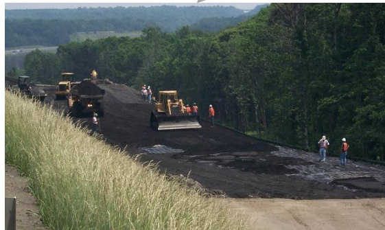
Road construction aggregate
