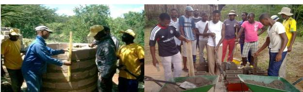
Around 300 blocks are used in the construction of a rondavel, and the block yard produces around 250 blocks a day.
