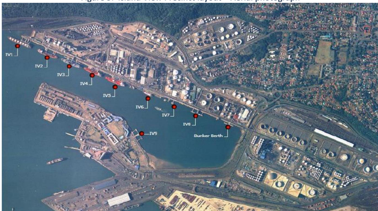
Figure 3: Island View Precinct layout – Aerial photograph
