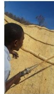
Applying water to soak the matting
