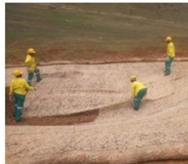
Laying the matting
